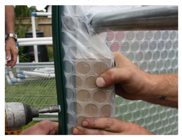
14.10 The Keder plastic is secured around the end hoop by being trapped between a length of 'Profile' and the hoop, and effectively clamped. One person will need to pull the plastic over the frame (using the noggin) keeping it tight, while the other person fits the profile into position using the Profile Screws (Rubber Washer) (ITEM 44). The Profile screws will drill their own holes, no pilot holes are required.
